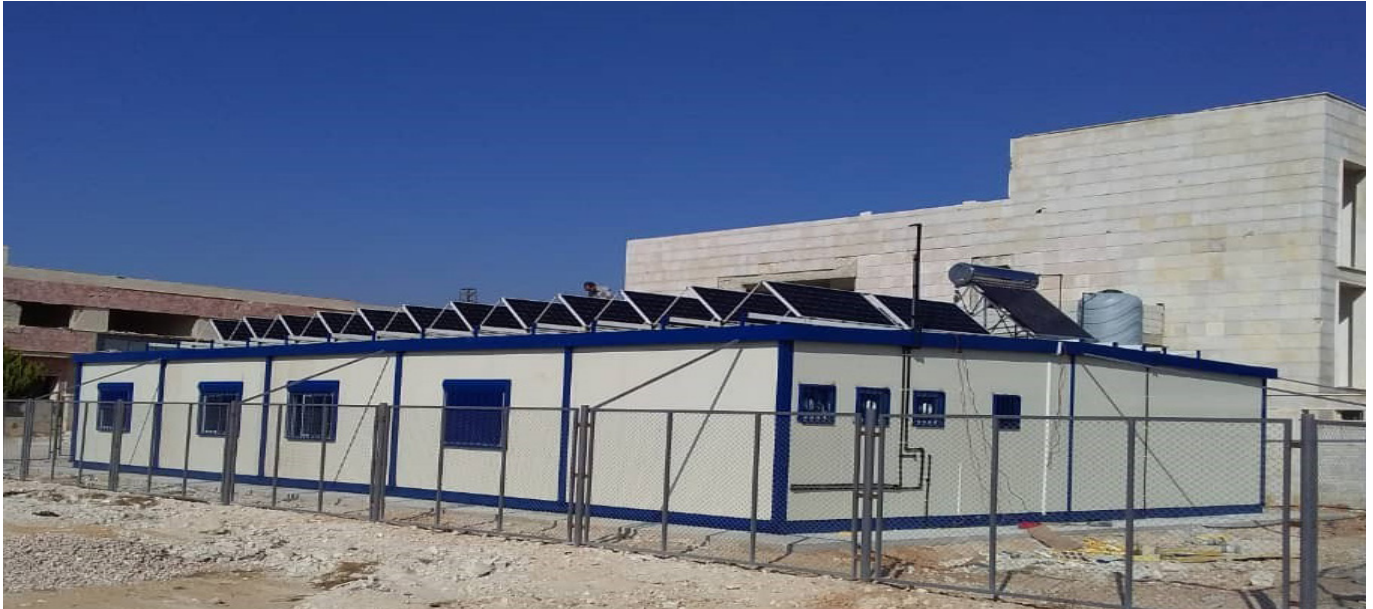
Prefabricated cadastral service center established in Qusayr city (UN-Habitat Syria)
