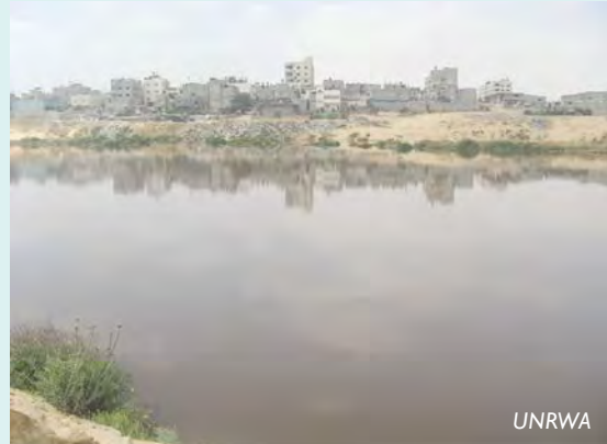
Sanitary drainage collection pond in Khan Younis as a result of the non-functioning of the sewerage network.
