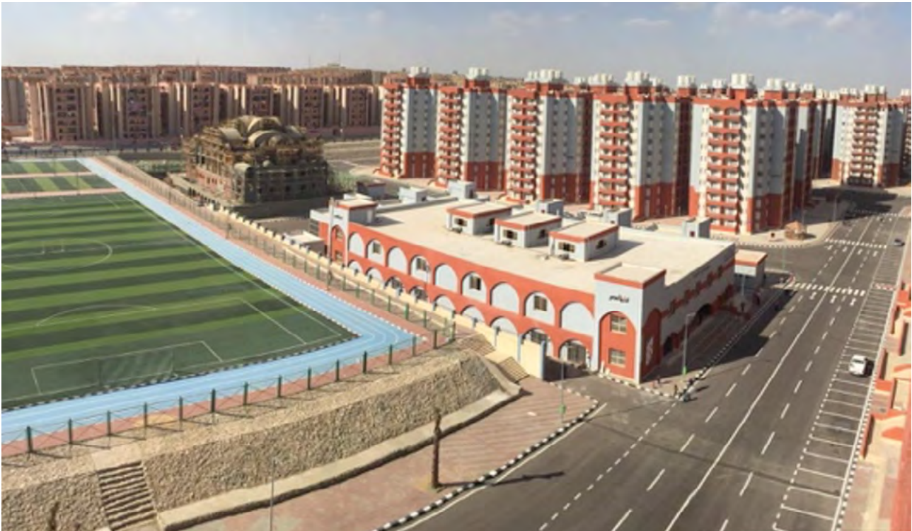
Figure III: Aerial view of El-Asmarat Source: (ElHanafi, 2019)
